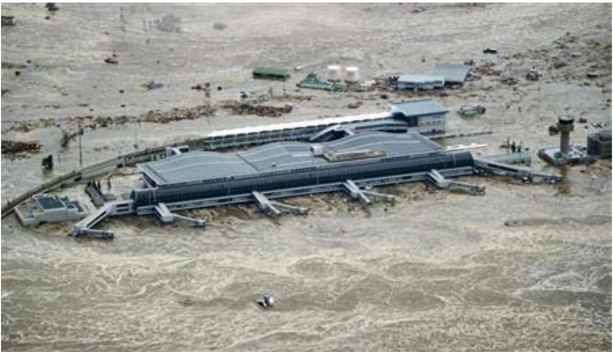
Figure 16 Sendai Airport when inundated by the tsunami. This is taken near the peak tsunami height (4–5 m). Source: Reuters.
