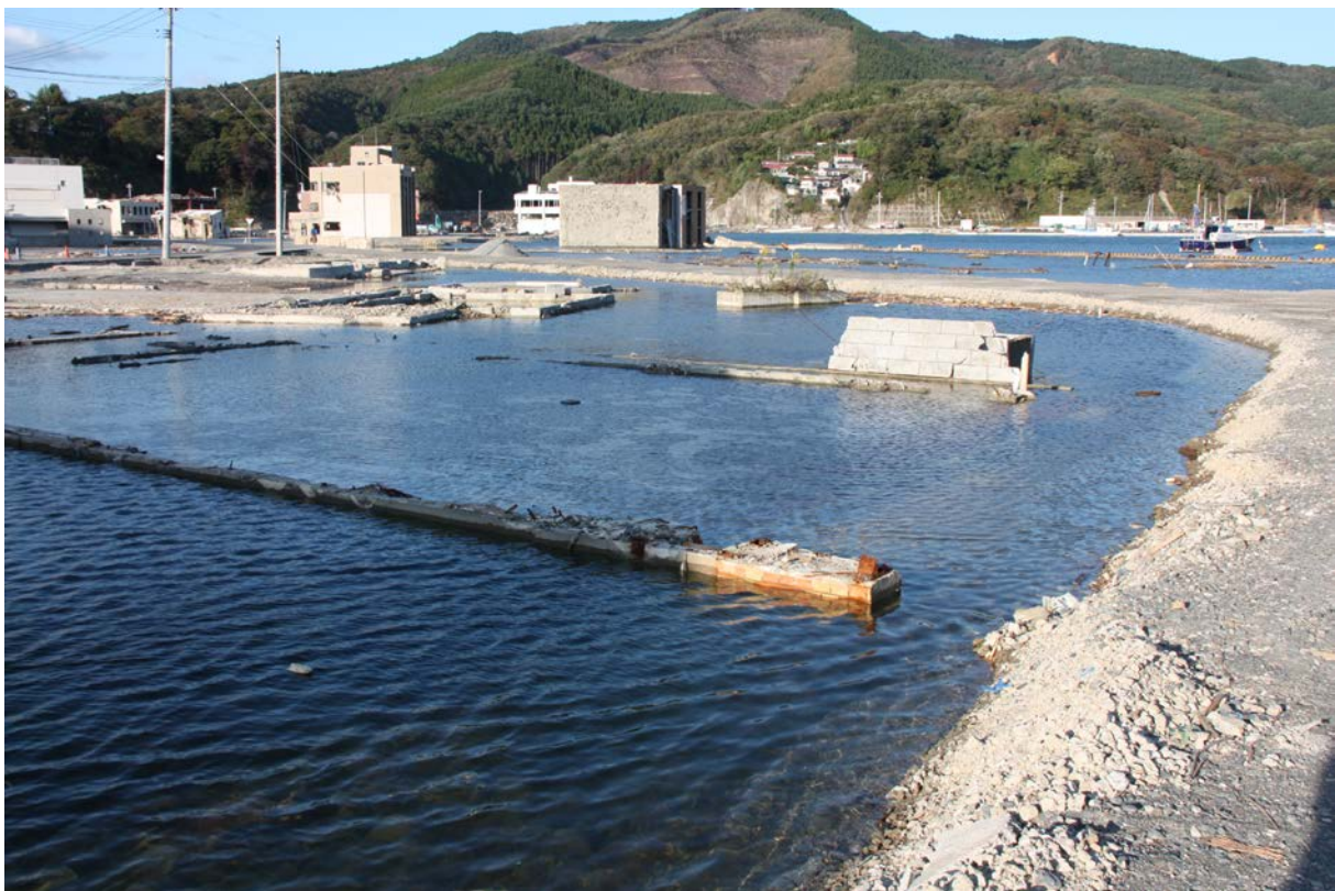
Figure 18 Subsidence reduced ground elevation, resulting flooding land in Onagawa, Japan. Taken six months after the Great East Japan tsunami, new roads have been constructed at a higher elevation. Source: S. Fraser and G.S. Leonard.
