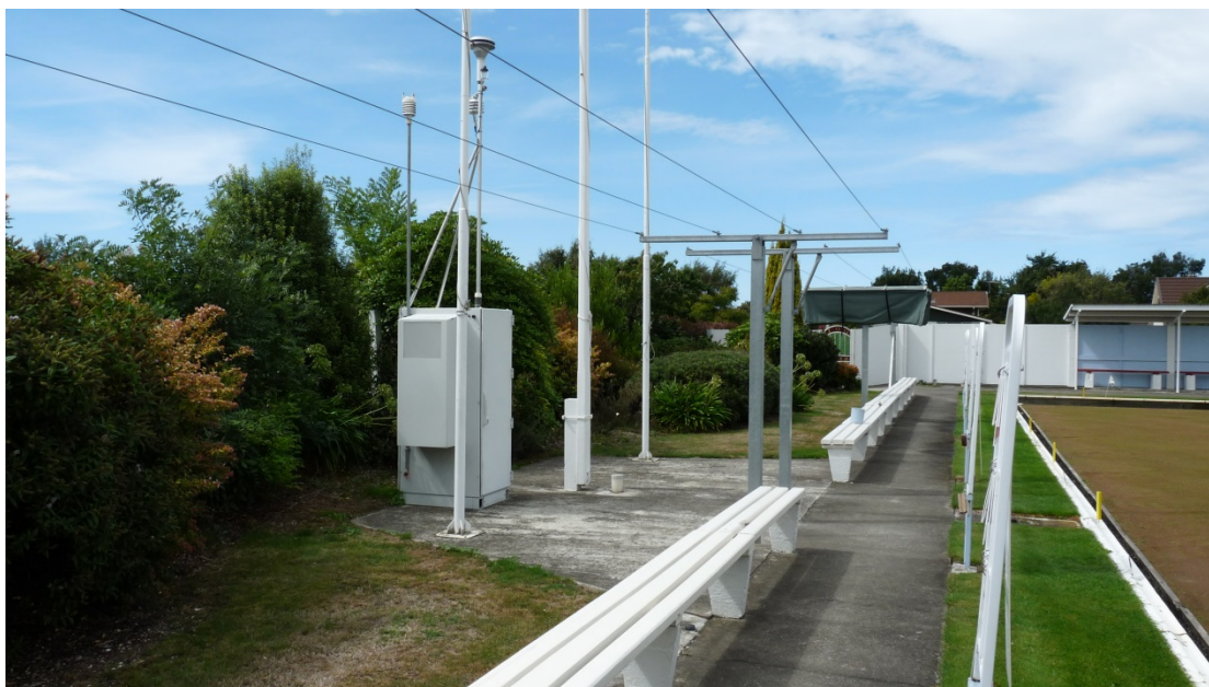
Figure 2.5: PM 10 monitor at the Redwoodtown – Bowling Club air quality monitoring site.
