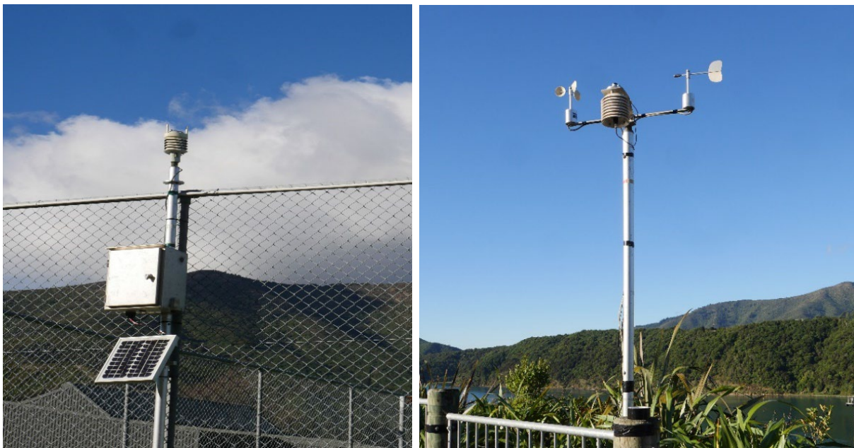
Figure 2-2: The two types of weather stations used in the study. Left is a Vaisala system and right is a Vector system.
