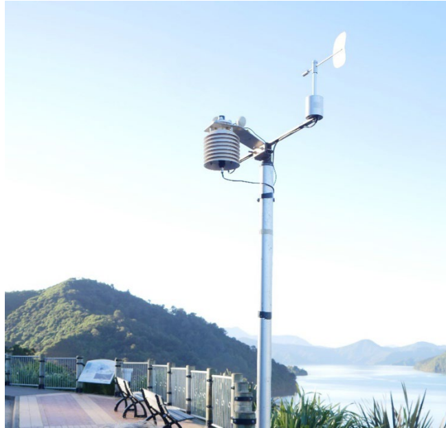
Figure A-9: Photo of the site looking to the NE.
