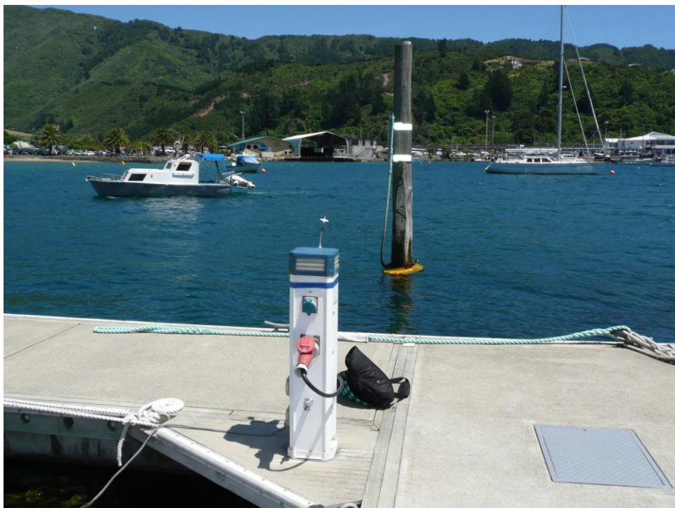
■ Figure 4: Picton Jetty PID Monitoring Site
