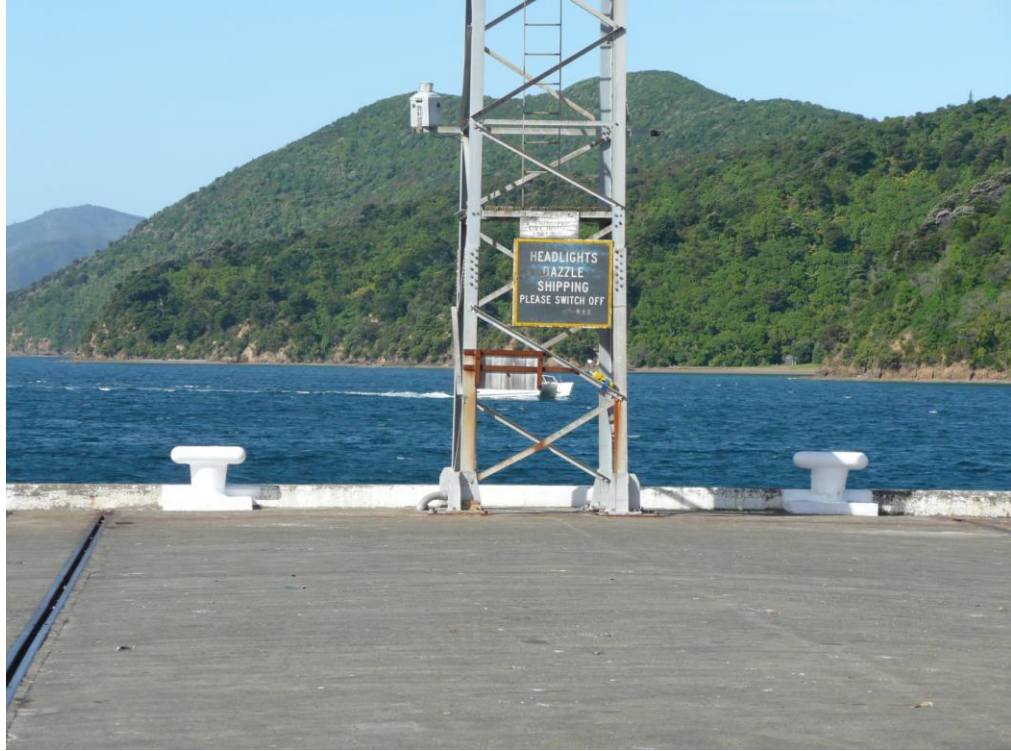
■ Figure 3: Waitohi Wharf PID Monitoring Site
