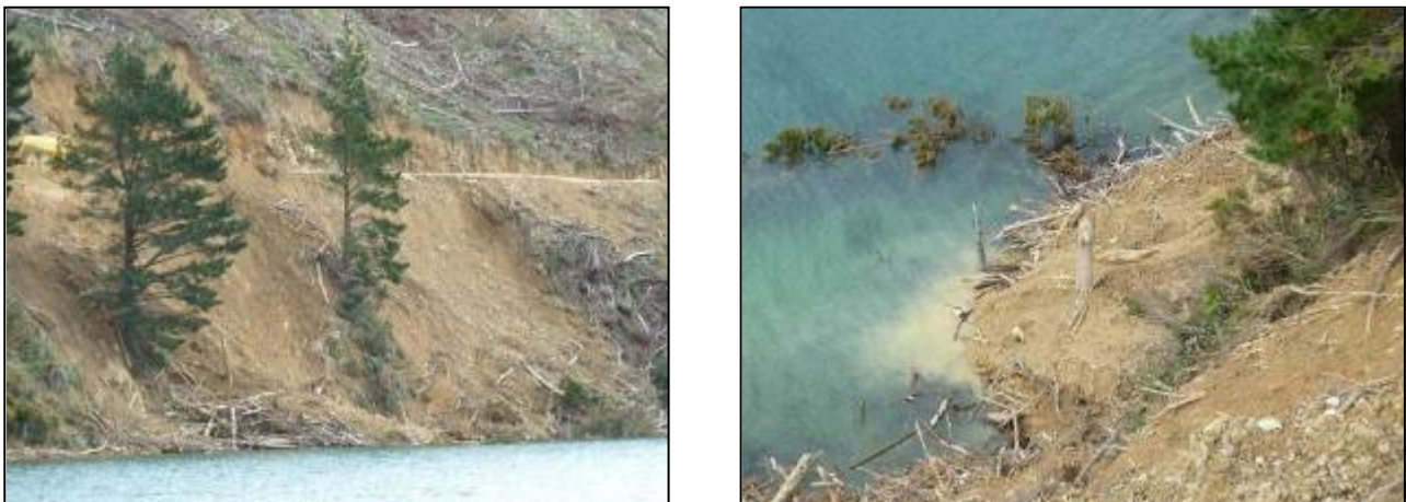
Figure 2: Instability of fill areas after road construction in Pelorus Sound 2012. Source: Marlborough District Council.
