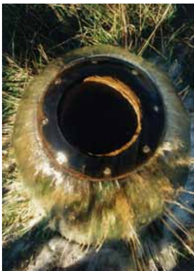
Figure 5.1: Naturally free flowing well 0403
