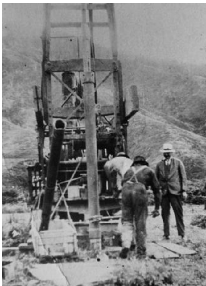
Figure 41.5: Water well drilling rig prospecting for gold at Cullensville 1924 (Marlborough Historical Society)
