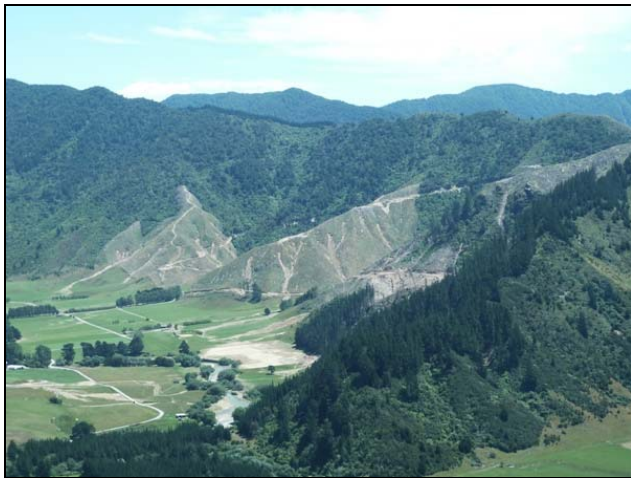
Figure A15 Site 15 a, erosion in recently harvested pine
