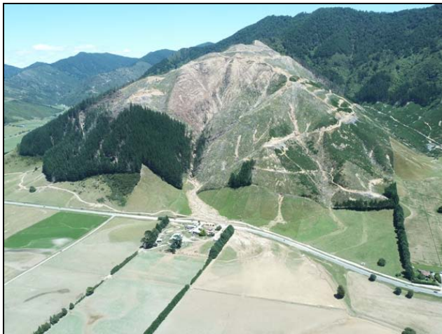
Figure A17 Site 17 a, b erosion in recently harvested pines
