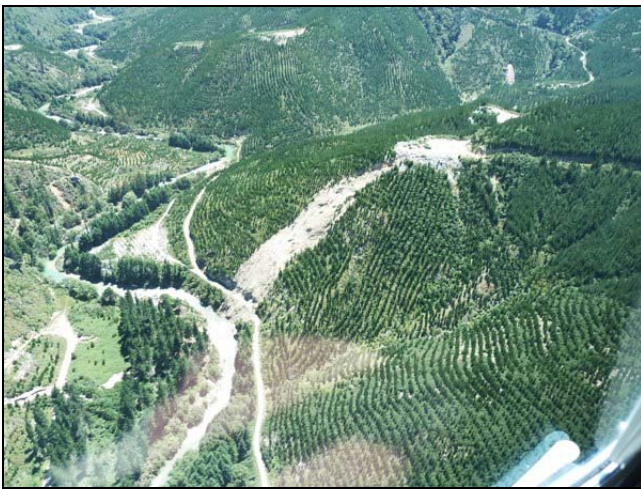
Figure A6 Site 6 erosion in pines <10 years
