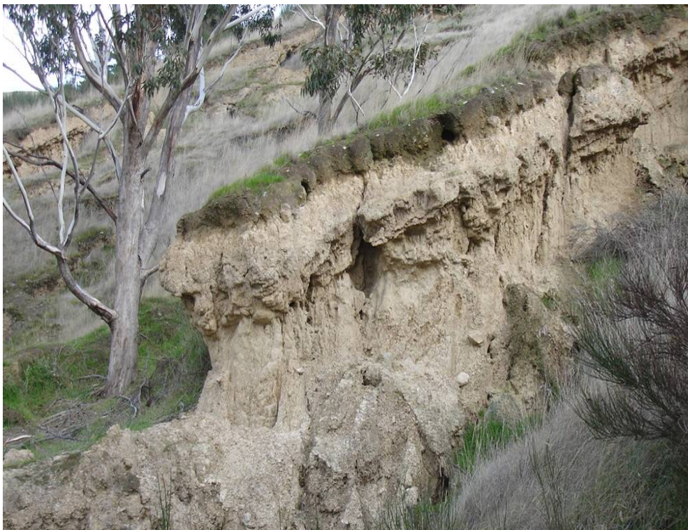
Figure 33. A piping channel forming below the fragic horizon in the dispersible clay loam, below a crack.
