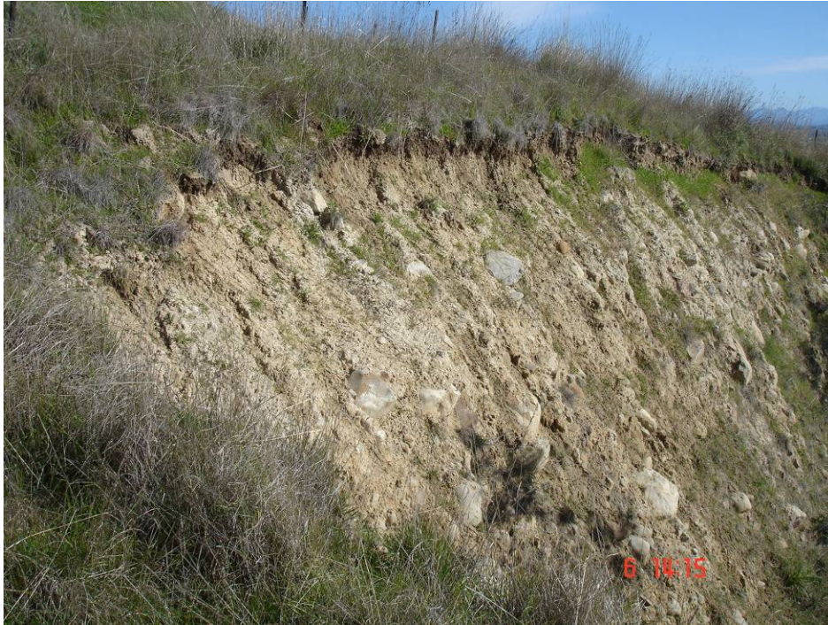
Figure 44. Vernon soils on deep lower slope deposits of loess and scattered boulders.
