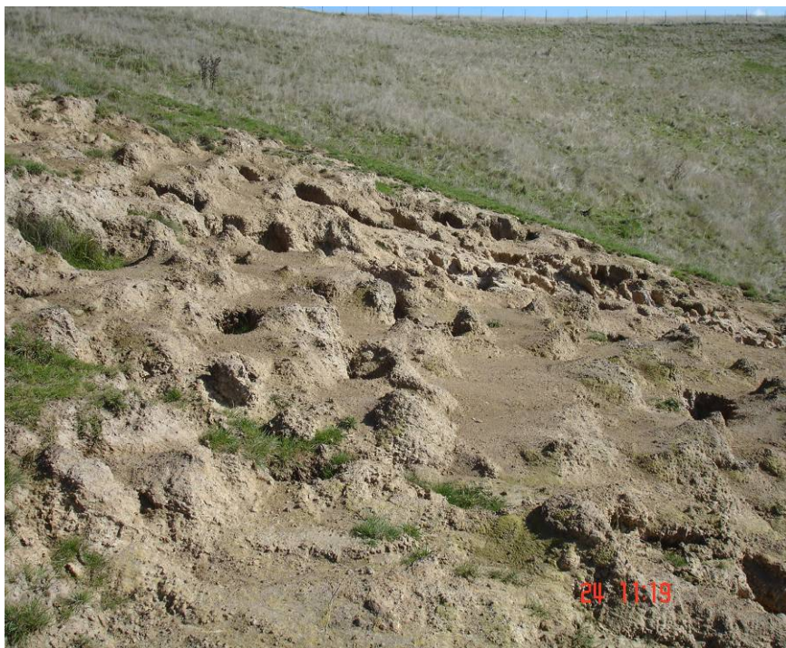
Figure 51. Extensive sheet erosion in a valley head site of Vernon hill soils.
