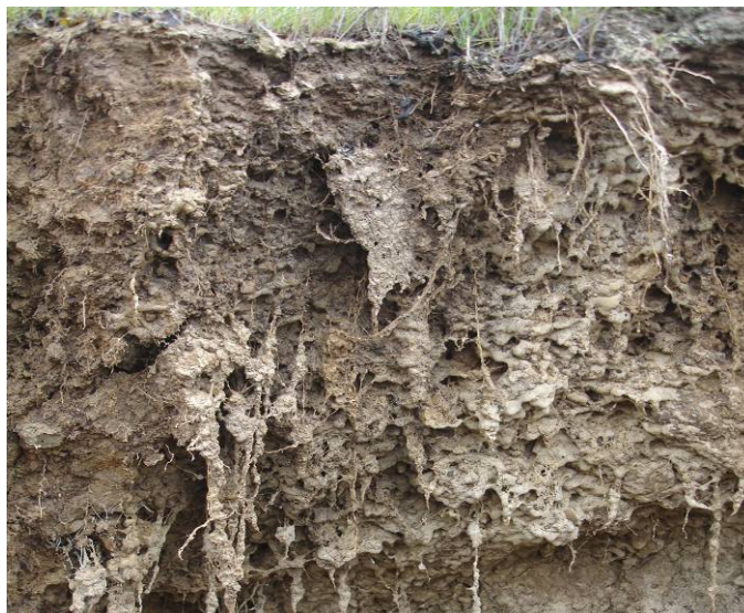
Figure 58. Surface soil material formed during mechanical gully infilling showing active dispersal. The dispersed soil either washes away in flood waters or may be re-deposited on lower slopes.
