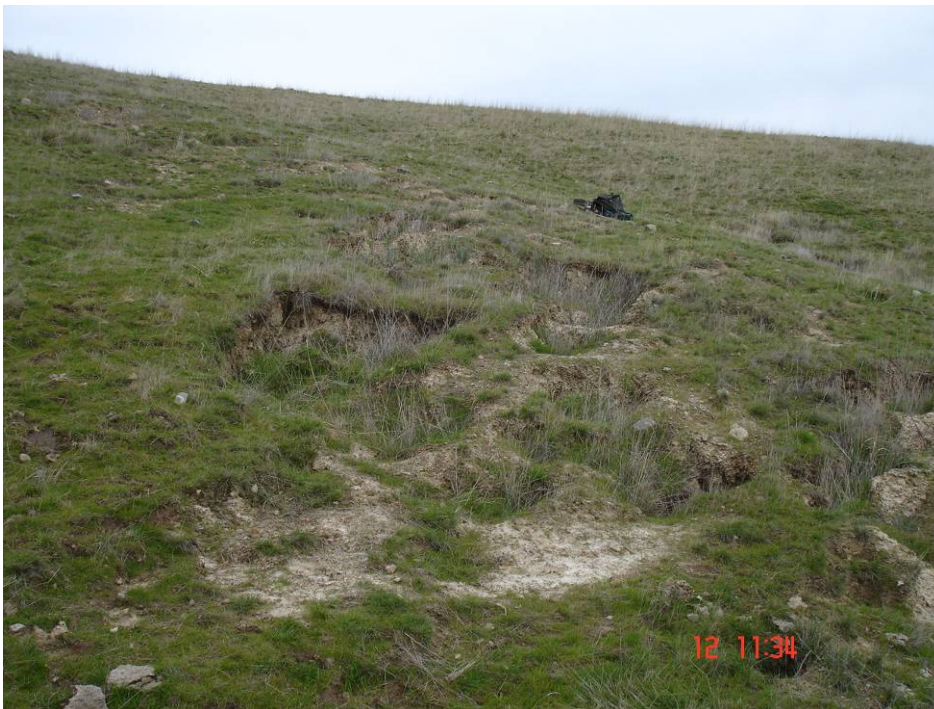
Figure 55. An area previously treated for erosion control with new gullies forming.
