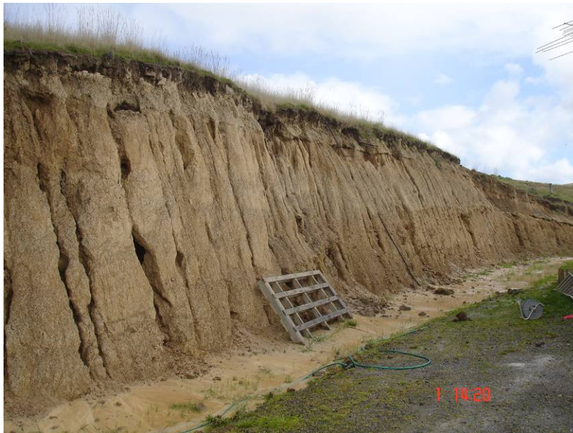
Figure 75. The building platform at this site is on stable underlying gravels. The layered dispersible loessial materials have scattered piping channels that will have originated somewhere up-slope. Rill erosion is taking place on the face of the cutting and dispersed soil sediment is accumulating at the foot of the cutting and being removed in suspension. The erosion will continue but is unlikely to pose a serious risk to the building structure. There is no evidence of mass movement (slumps) occurring in these materials.
