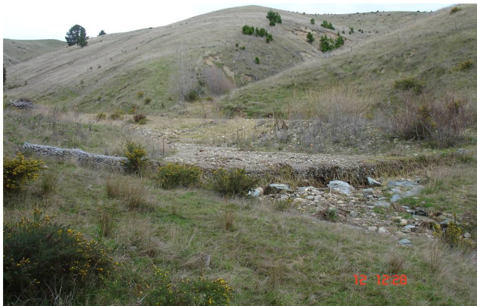
Figure 72. A sediment retention dam built by the Marlborough Catchment Board as part of erosion control measures. Impounded sediments are periodically removed to maintain the sediment retention function, but a better alternative might be to build a new structure on top of the retained sediments.
