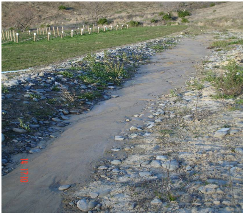
Figure 70. This runoff diversion barrier has trapped a small amount of silt and emphasises the ongoing loss of fine soil material from adjacent hill and steep slopes. Without the barrier, the silt would have ended up in the waterways of the Wairau Plain.
