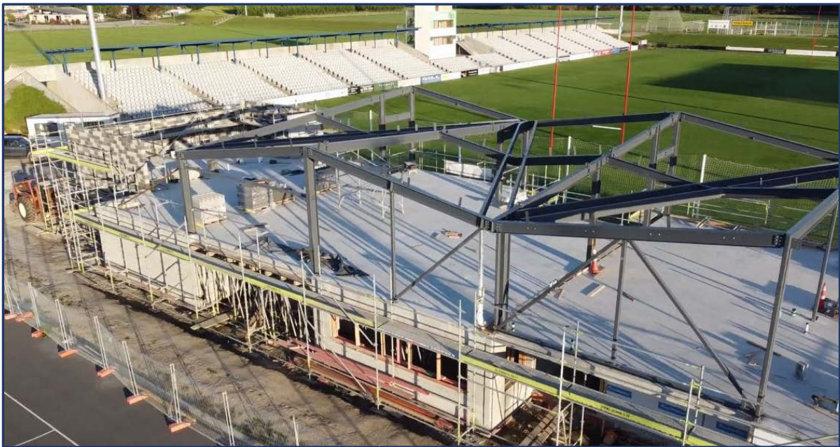
Lansdowne Hub under construction
