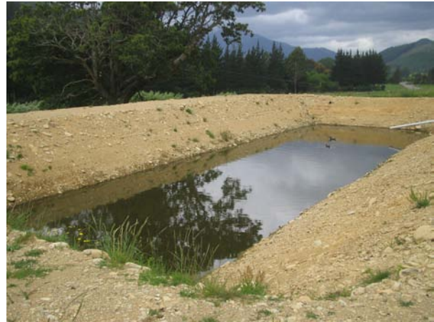
Pond managed so that there is capacity to store effluent during rain events
