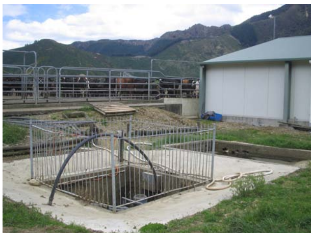
Although not a resource management requirement, sumps and ponds should be fenced for safety reasons
