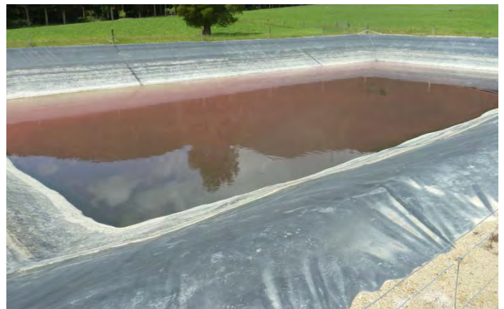
Effluent pond has plenty of free-board available
