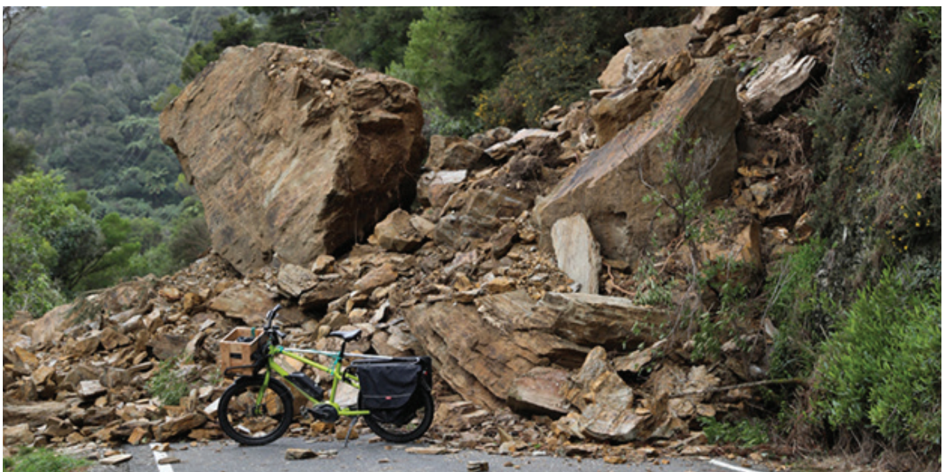
Slip on Kenepuru Road, credit BP Fisher
