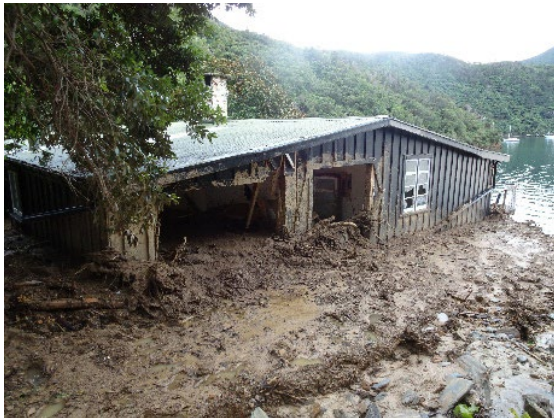
DS4 – Severe: Irreparable structural damage
