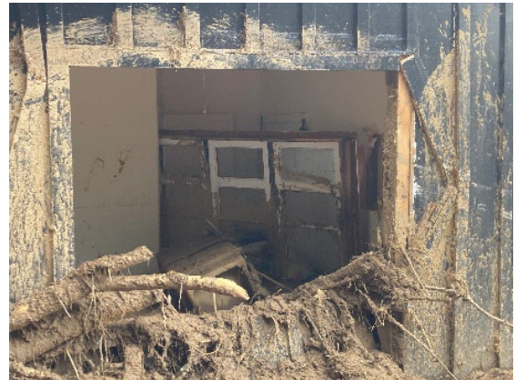
DS4 – Severe: Irreparable structural damage
