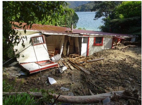
DS5 – Critical: Structural integrity fails
