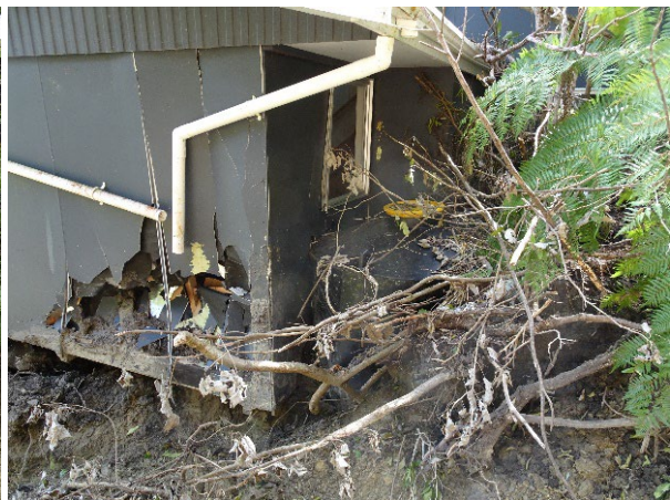
DS2 – Light: Non-structural damage only
