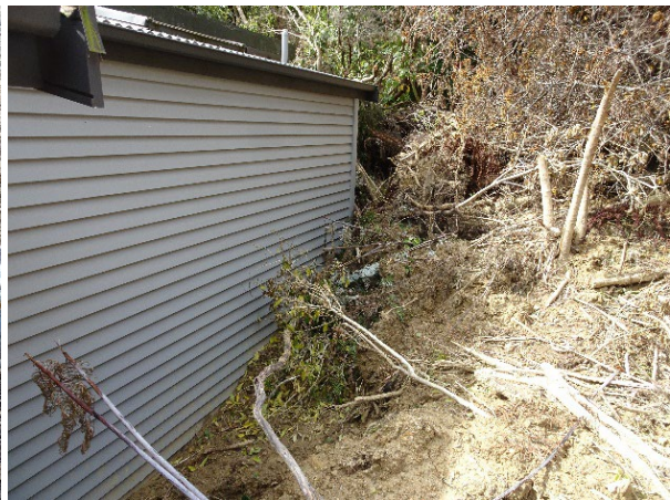
DS1 – Insignificant: Minor non-structural damage
