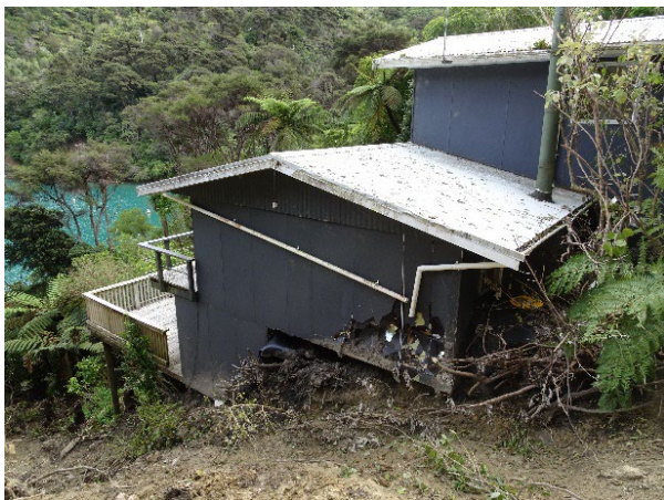
DS2 – Light: Non-structural damage only
