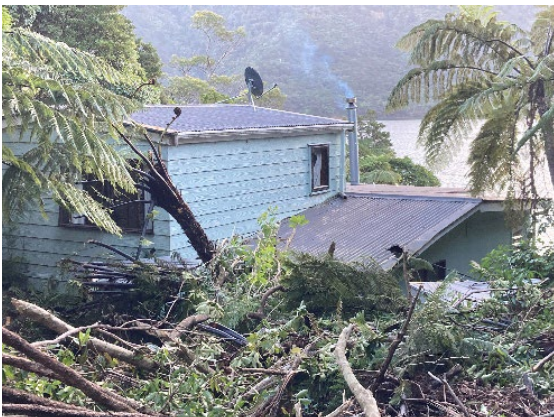
DS2 – Light: Non-structural damage only
