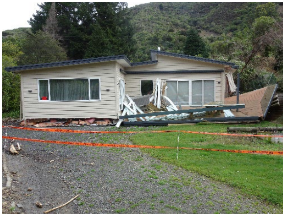
DS5 – Critical: Structural integrity fails
