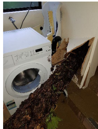
DS2 – Light: Non-structural damage only
