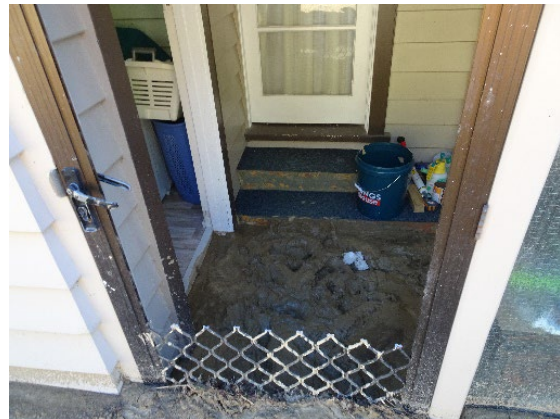
DS1 – Insignificant: Minor non-structural damage
