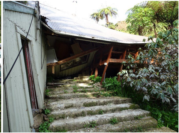
DS5 – Critical: Structural integrity fails
