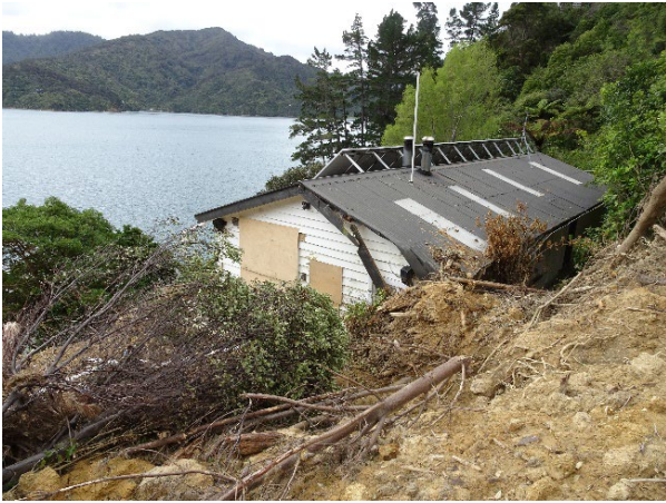
DS3 – Moderate: Reparable structural damage
