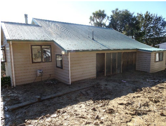
DS1 – Insignificant: Minor non-structural damage
