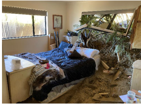
DS3 – Moderate: Repairable structural damage
