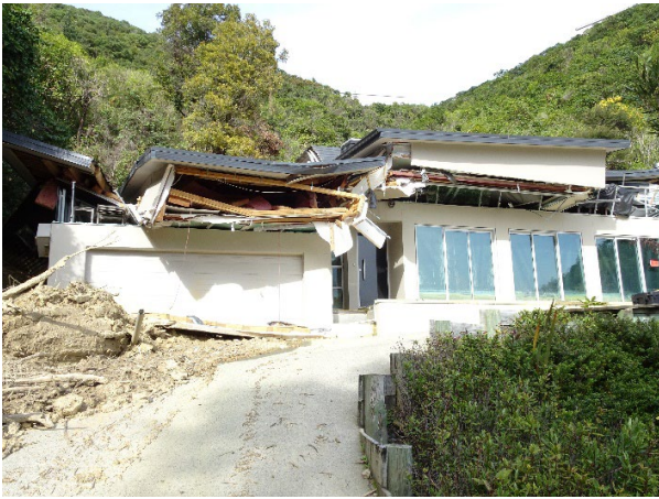
DS5 – Critical: Structural integrity fails
