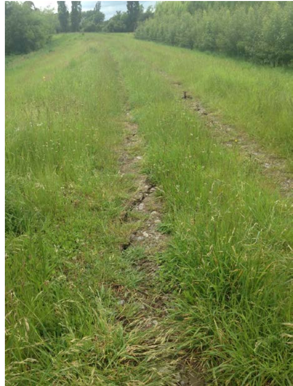
Figure 2 - Surface cracking of LW06 caused by lateral spread from the 2016 Kaikōura earthquake
