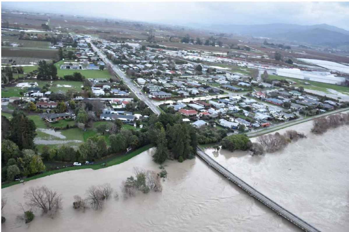
Figure 8 - July 2021 flood event showing LW05 on the right side of the photo close to design limit with minimal flood capacity safety margin (freeboard) remaining, photo taken at the peak of the flood
