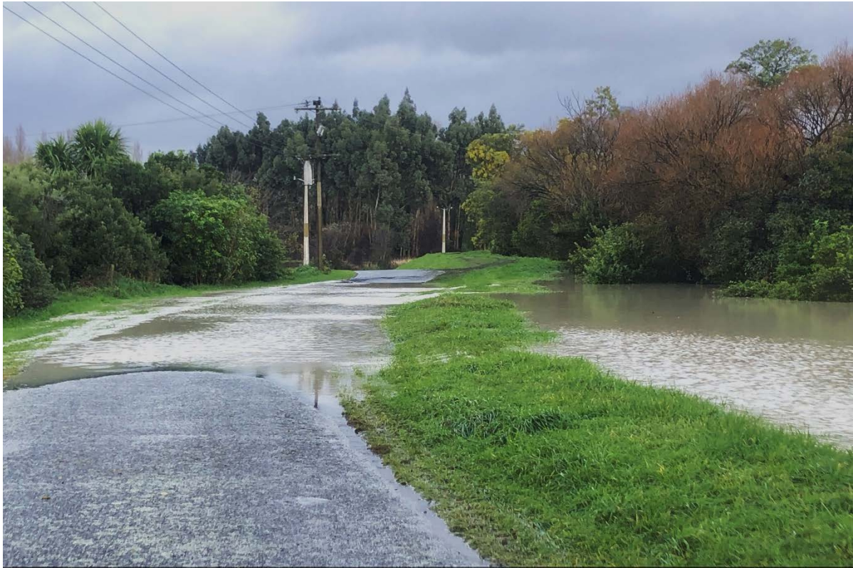
Figure 7 – July 2021 flood event showing LW05 still overtopping an hour after the peak of the flood. Scour damage to the rear face of the bank occurred as a result – the first stage in an overdesign event bank failure
