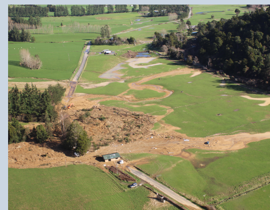
📷 A house in the middle of Ronga Road after the August 2022 storm
