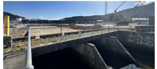
Waitohi Culvert works underway
