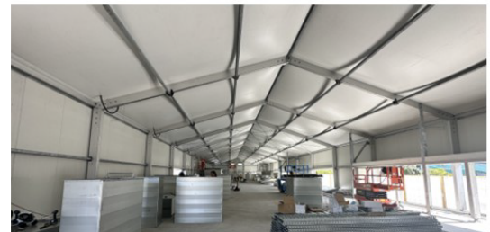
Temporary Terminal Building Construction underway
