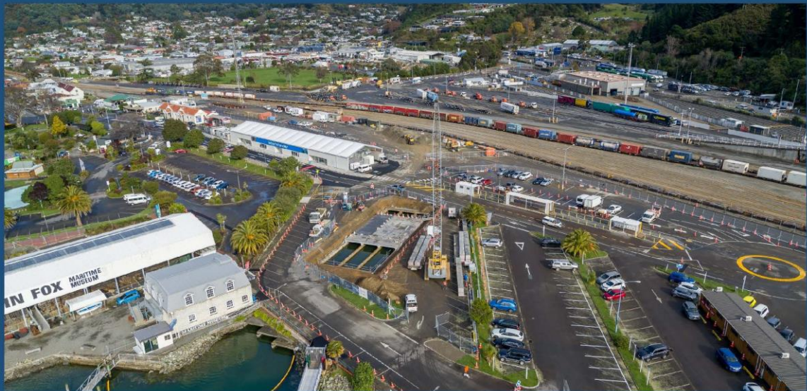
Waitohi Culvert Upgrade
