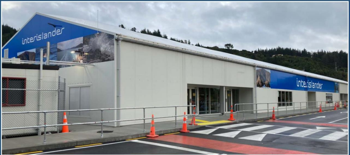
Temporary Terminal Construction - Complete
