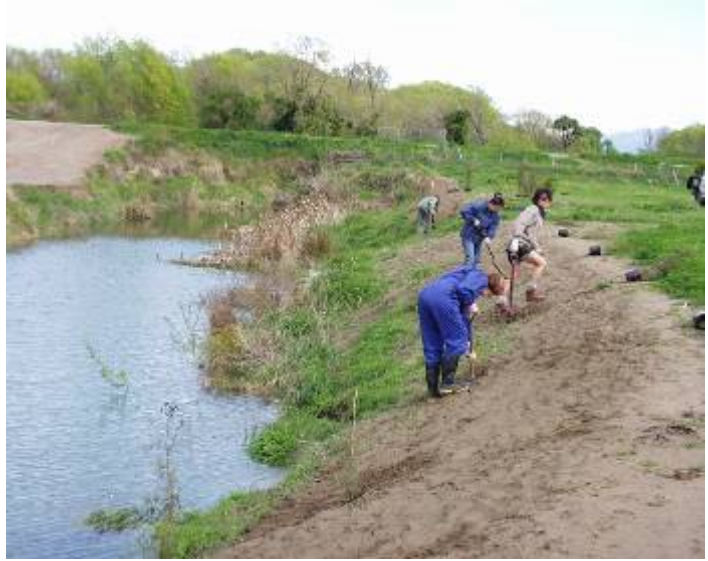
Planting northern outlet of Grovetown Lagoon
