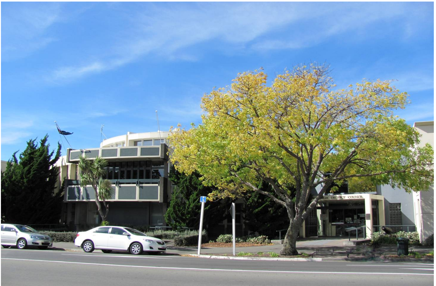
Picture: Marlborough District Council building, Blenheim
