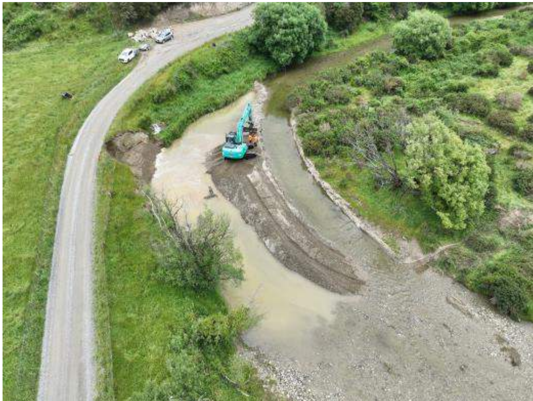
Diversion works ready for rock protection placement on Waikakaho Road
