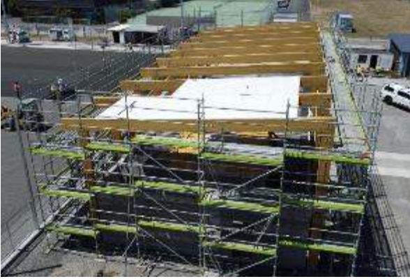
Fig. 5 – Hockey Pavilion, roof installation underway.
