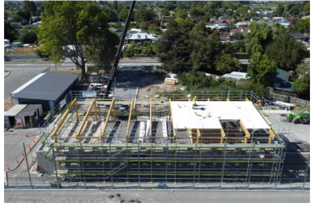
Fig. 6 – Hockey Pavilion, roof installation underway.
