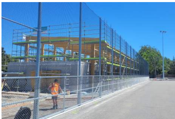
Fig. 2 – Hockey Turf, south high ball fence completed.
