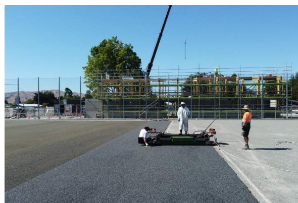
Fig. 4 – Hockey Turf, Ecocept underlay installation.
