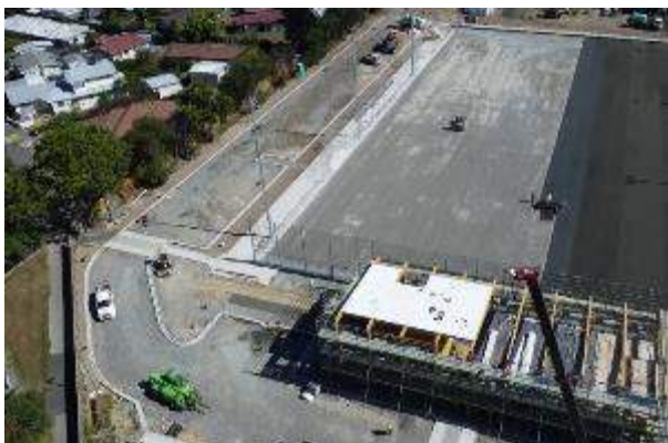
Fig. 1 – Hockey Turf, car park construction.
