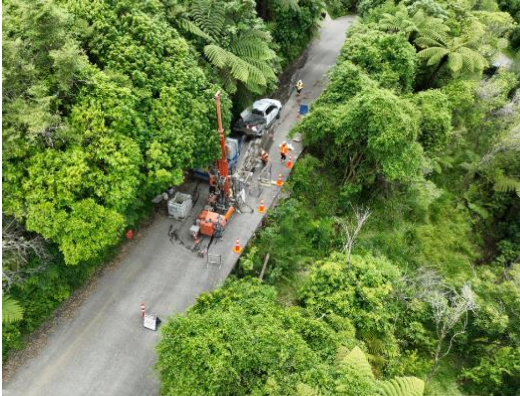
Drilling work occurring on Tepuia Heights Road
