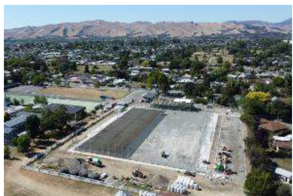
Fig. 3 – Hockey Turf, Ecocept underlay installation.
