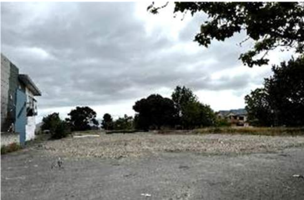
Fig. 7 – 6 Russell Terrace, demolition complete.
