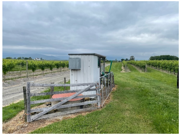
P4: Pump shed.
