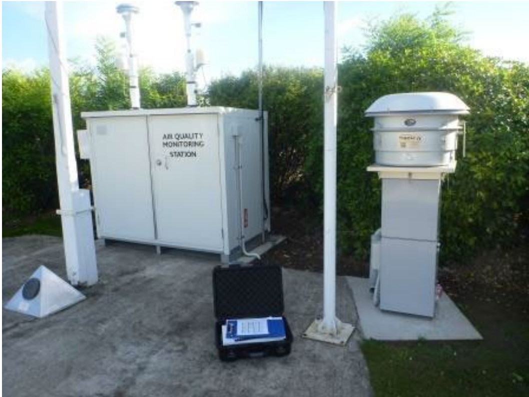
Figure 2.3: PM 10 monitor at the Redwoodtown – Bowling Club air quality monitoring site.
