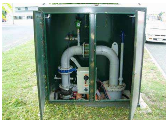
Figure 1.5: Municipal well-field at Grove Road in central Blenheim
