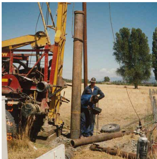
Figure 6.4: New section of casing being added.
