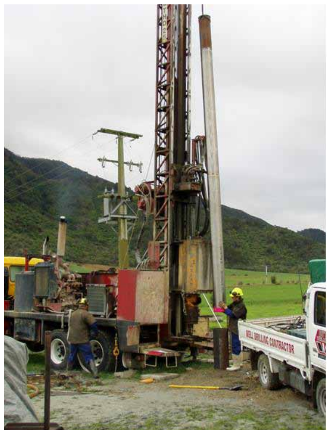
Figure 6.11: Long screen at Parkes well Linkwater
