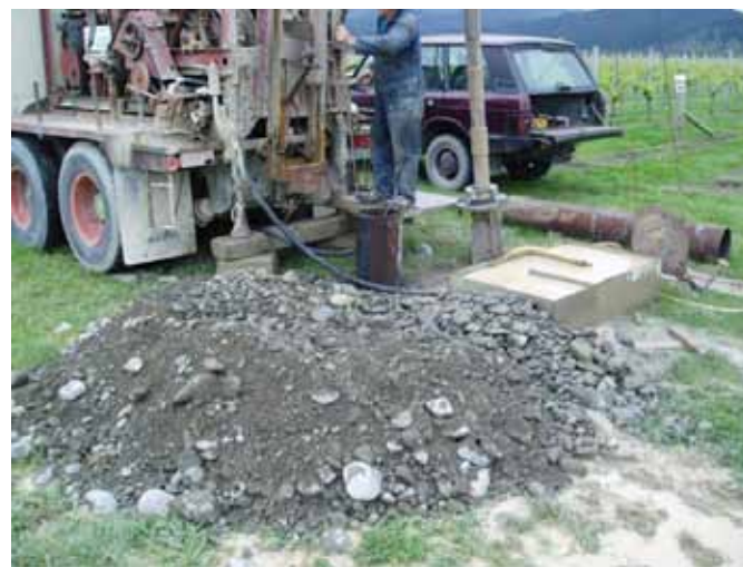
Figure 6.2: Cable tool resting on the ground to the right of the driller, Colin Simpson during construction of Renwick municipal wellfield 2008
