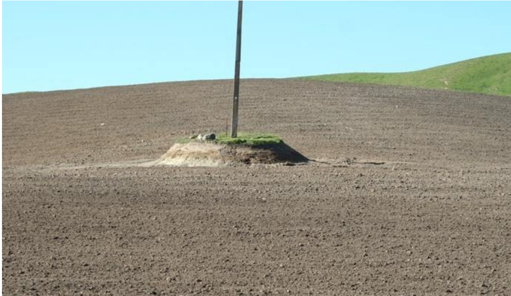
Fig. 1 Significant earthworks are involved in much of the landscape recontouring for viticulture currently being undertaken in Marlborough. An example of at least 1 m of ground surface lowering, south of Seddon; Grid reference: 2601660E; 5943426N. (Photo: Colin Gray, Marlborough District Council)
