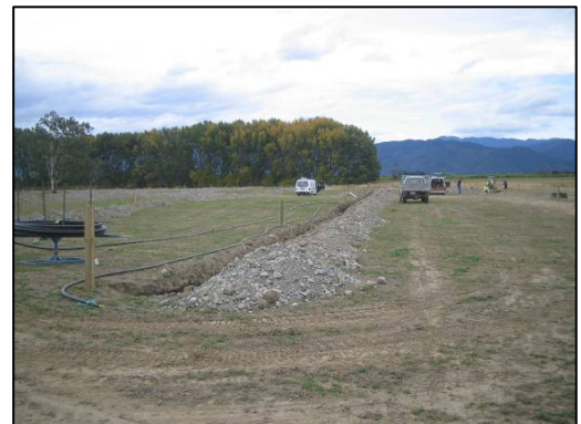
Installation of a 9 hectare disposal area
