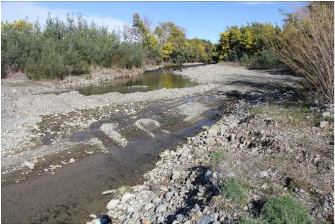
Figure 2: Diversion 3 with flow seeping through the gravels
