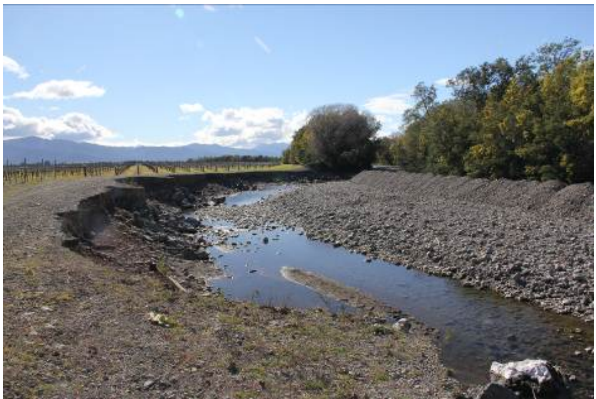
Figure 1: Diversion 2 showing remaining flow seeping through the gravels.
