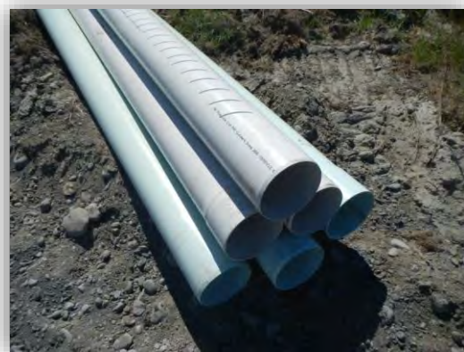
Figure 12: Gallery conduit with machine cut perforations
