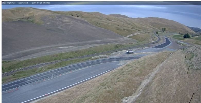
Dashwood Alignment looking south; Tuesday 25 Nov 2014.
