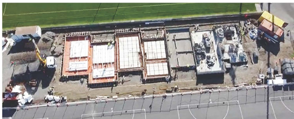
Aerial image of the concrete slab being poured
