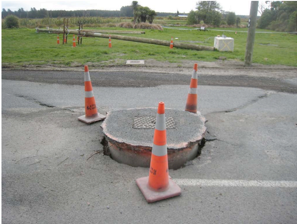
Figure 29. Floated Sewer Manhole, Brooklands (one of fifteen)
