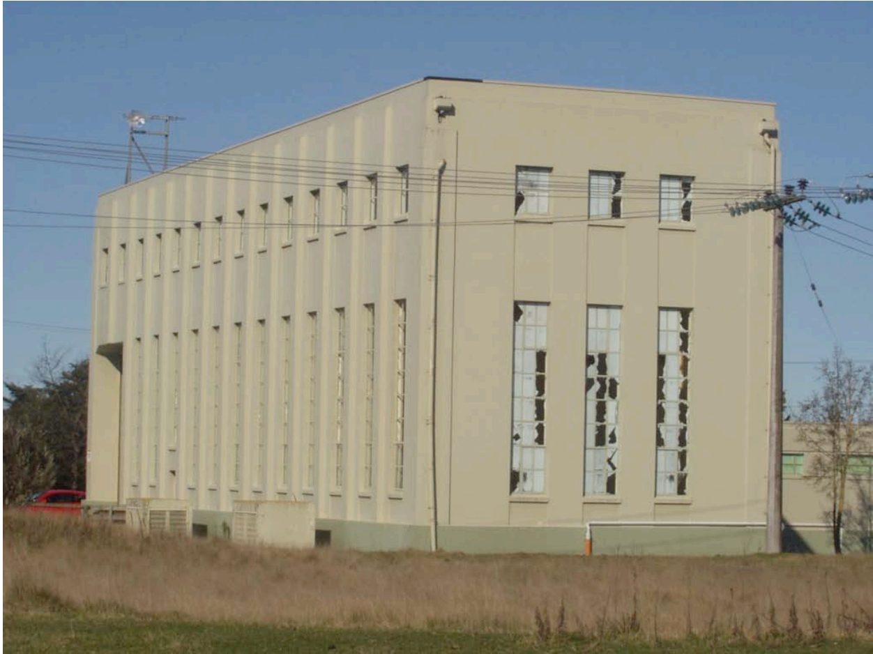
Figure 17. Hororata Control Building
