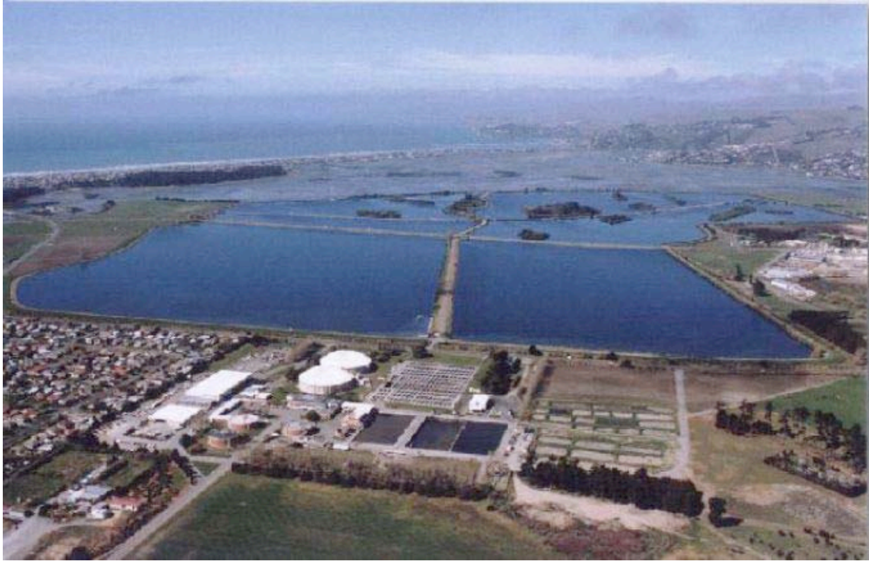
Figure 26. Christchurch CWTP at Bromley
