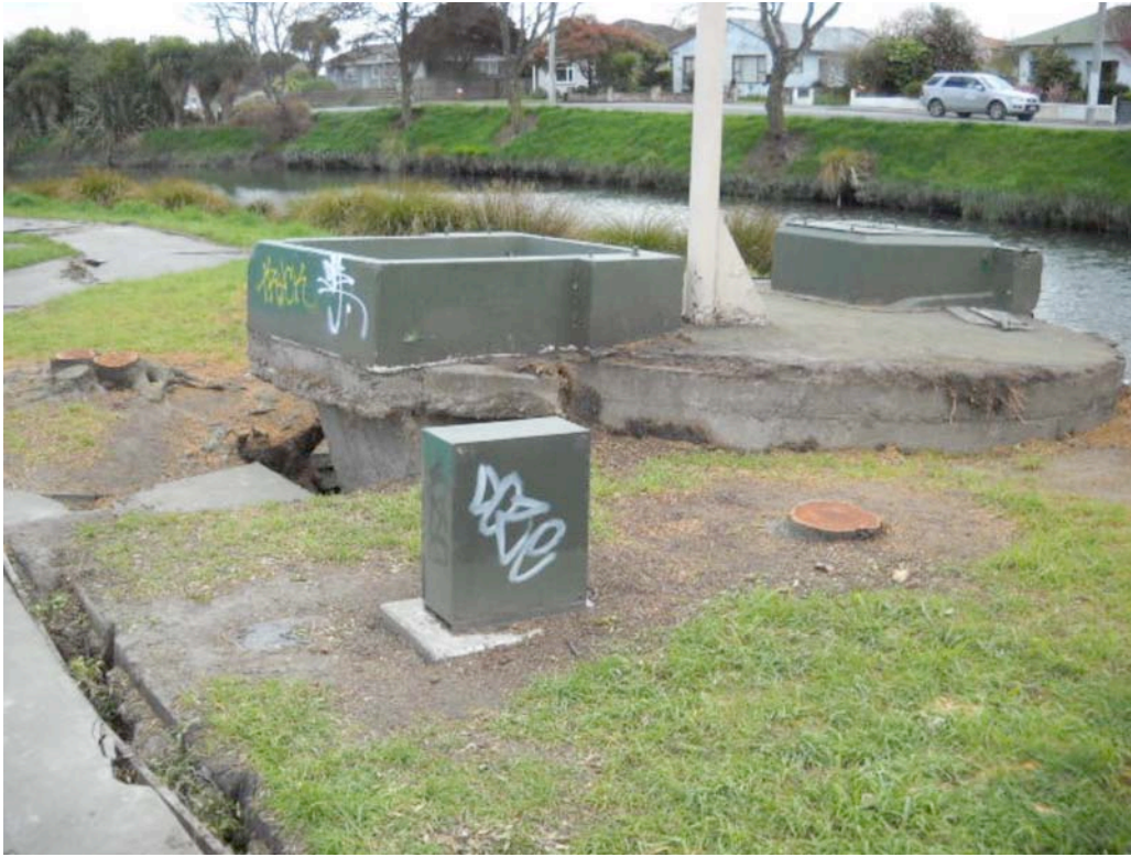
Figure 28. Floated and Tilted Wastewater Life Station 27, Avonside
