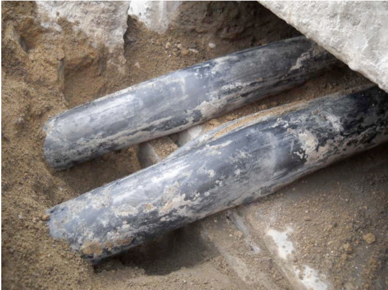
Figure 22. 66 kV Cables
