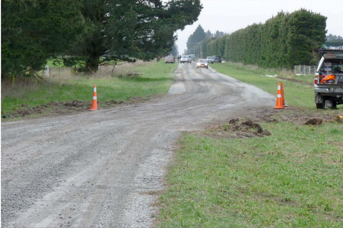
Figure 8. Fault Offset Through a Road
