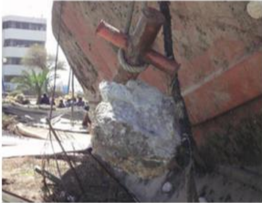
Figure 11. Uprooting of a steel-concrete mooring in Talcahuano, Chile, after the 27 th February 2010 Chile. Source (Palermo et al. 2013)
