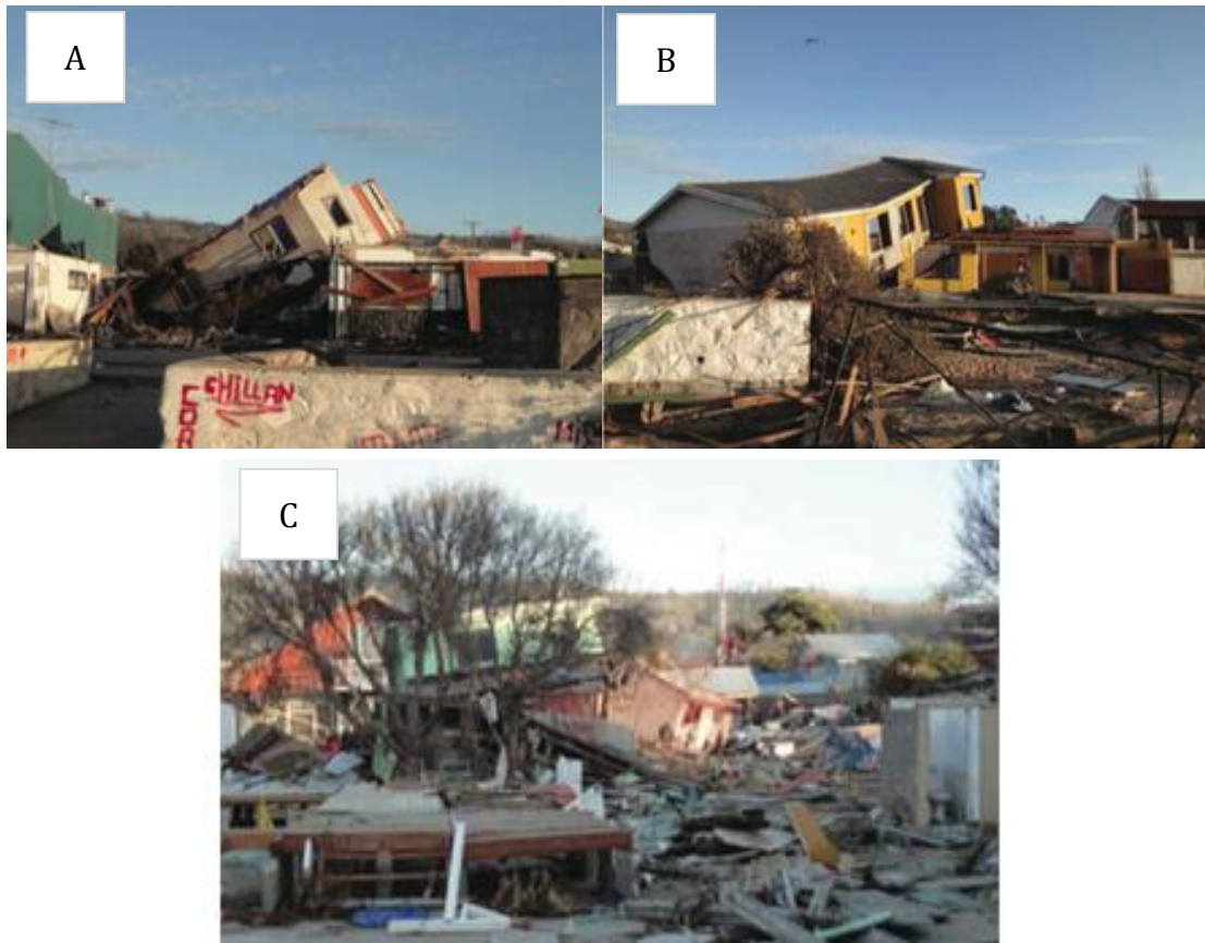
Figure 8. (A-B) Sliding and unseating of storey levels in Dichato, Chile after the 27 th February 2010 Chile Tsunami. Source (Palermo et al. 2013) (C) Widespread damage timber homes in Dichato, Chile after the 27 th February 2010 Chile Tsunami resulting in extensive timber debris. Source (Palermo et al. 2013)
