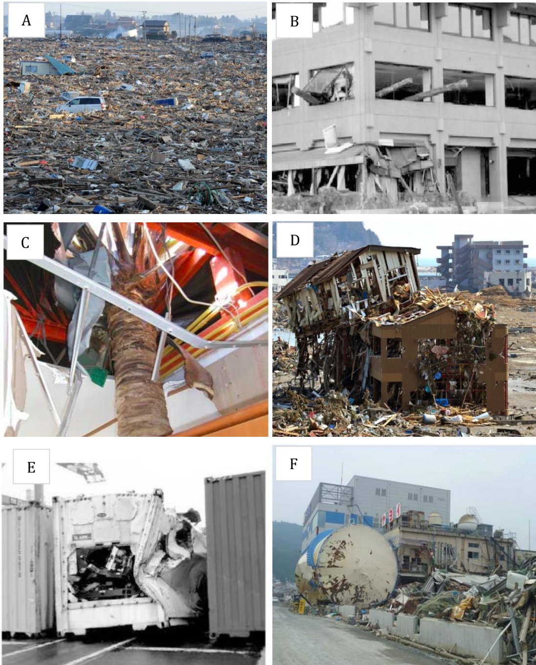
Figure 4. (A) Extensive mounds of debris in Natori, Miyagi prefecture, Japan after the 2011 Japan tsunami. Source ( http://www.ibtimes.co.uk/2011-earthquake-tsunami-60-powerful-photos-disaster-that-hit-japan-five-years-ago-1548255 ). (B) An example of timber log debris in port buildings at Ofunato, Japan after the 2011 Japan tsunami. Source (Chock et al, 2013). (C) A coconut palm tree entrained by the December 26 th 2004 Tsunami, see here penetrating through a roof and internal ceiling of a hotel room on Koh Phi, Thailand. Source (Bell et al. 2005). (D) A building has become unseated from its foundations and been transported in the flow as large and potentially damaging debris and finally rested ontop of another building in Minamisanriku, Miyagi prefecture, Japan. Source ( http://www.ibtimes.co.uk/2011-earthquake-tsunami-60-powerful-photos-disaster-that-hit-japan-five-years-ago-1548255 ). (E) An example of damage to the debris (shipping container) due to strikes with other containers or structures. Source (Chock et al. 2013). (F) . A damaged storage tank that has been removed and transported from its original position in Kesenuma, Japan, during the Great East Japan Tsunami. Note the buckling and/or impact damage to the side of the tank nearest the road. Source (Horspool et al. 2016).
