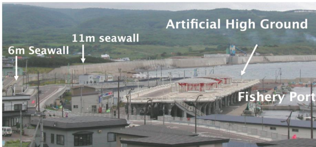
Figure 7. Artificial high ground in a fishery port. Workers can work daily on the first floor and use the second floor for evacuation purposes during a tsunami. Source (PIANC. 2010)
