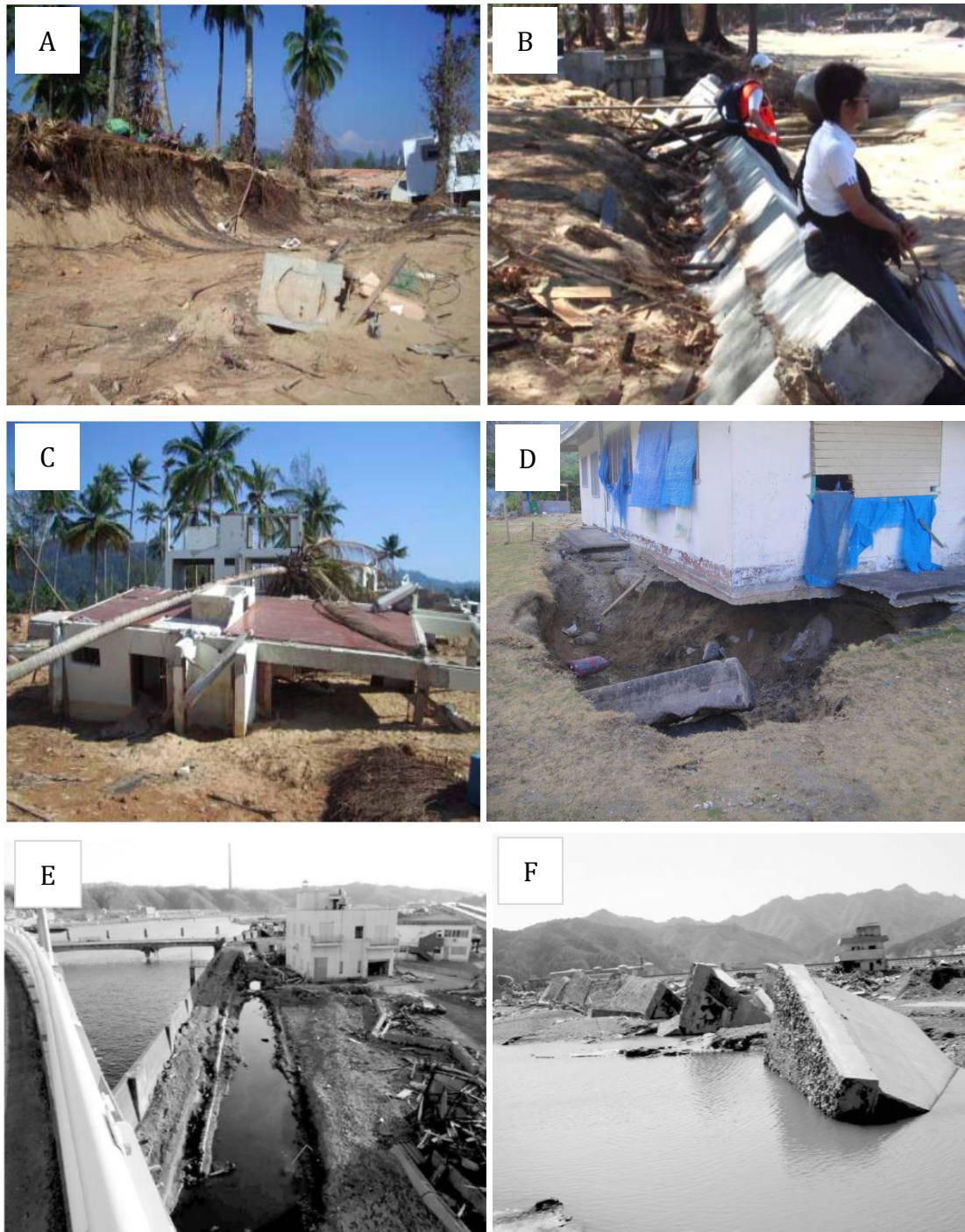
Figure 3. (A) Receding waters after waves from the 26 th December 2004 tsunami scoured channels with dimensions up to 50m wide and up to 3m deep shown here, in Khao Lak, Thailand. Source (Bell et al. 2005). (B) Receding waters from the December 26 th 2004 tsunami causing the collapse and tilting of most seawall defences on the Andaman Coast, Southern Thailand due to scouring on the landward side. Source (Bell et al. 2005). (C) Extensive scour from the 26 th December 2004 tsunami completely undermining nearby resort buildings in Khao Lak, Thailand, source (Bell et al. 2005). (D) Tsunami induced scour around the corner of buildings in Masefau, American Samoa during the 2009 Samoa tsunami. Source ( https://walrus.wr.usgs.gov/news/samoareports.html ). (E) Scour trench formed on the landward side of a flood wall in Miyako, Japan after the 2011 Japan tsunami. Source (Chock et al. 2013). (F) Damage to a concrete gravity seawall with shallow foundations in Otsuchi Port, Japan, due to a deep scour trench forming on the landward side of the structure, resulting in collapse and dispersal of monolithic concrete blocks up to 70m inland. Source (Chock et al. 2013).
