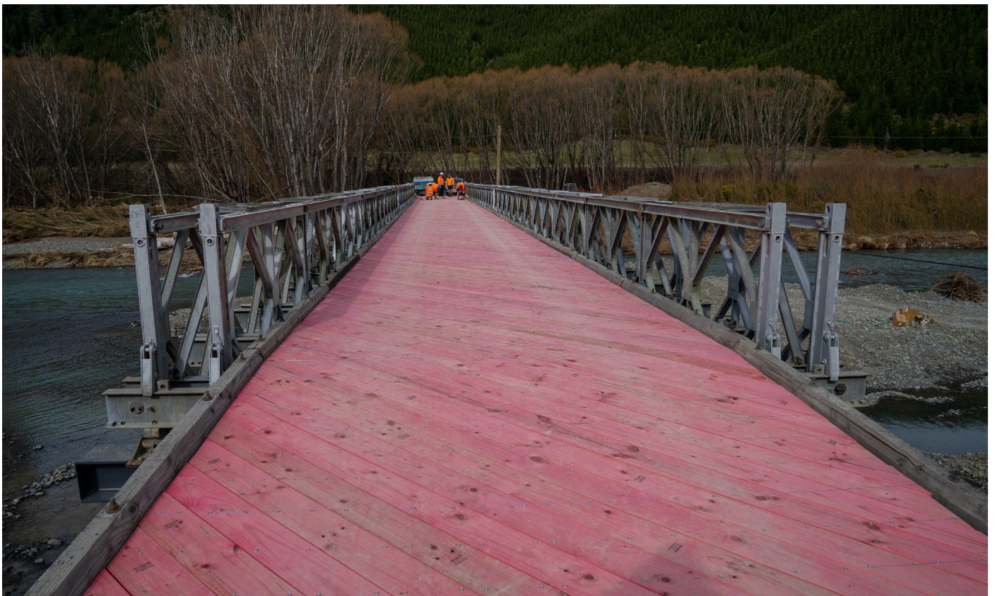
The temporary Bailey bridge to replace the Māori Ford Bridge in the Waihopai Valley which was swept away
