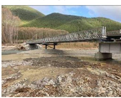
Waihopai (Bailey Bridge)
