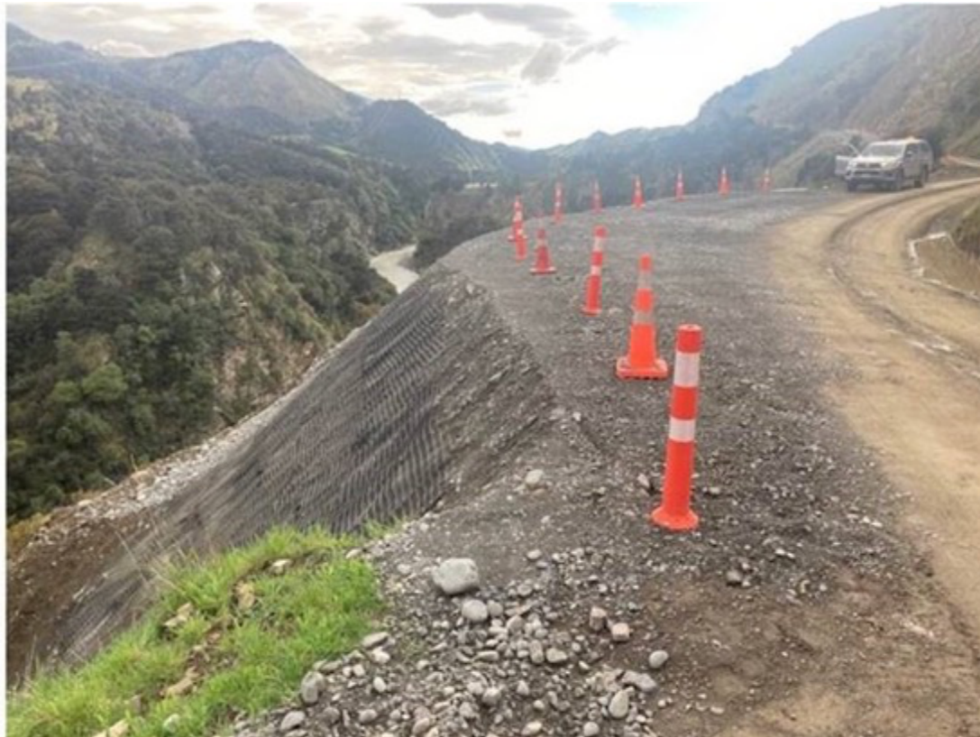
Awatere Valley Road – completed slip repair at RP 7740
