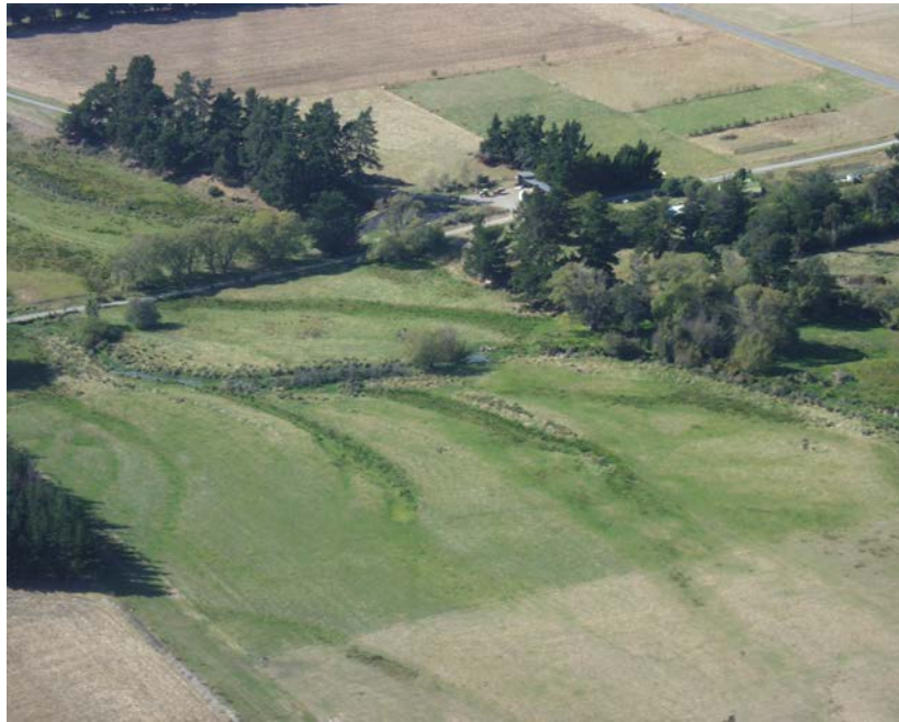
Figure 4: Groundwater convergence at Mill Road feeding into a south tributary of Mill Stream. Site MST-26 is located at the road culvert on the middle right of the photo.
