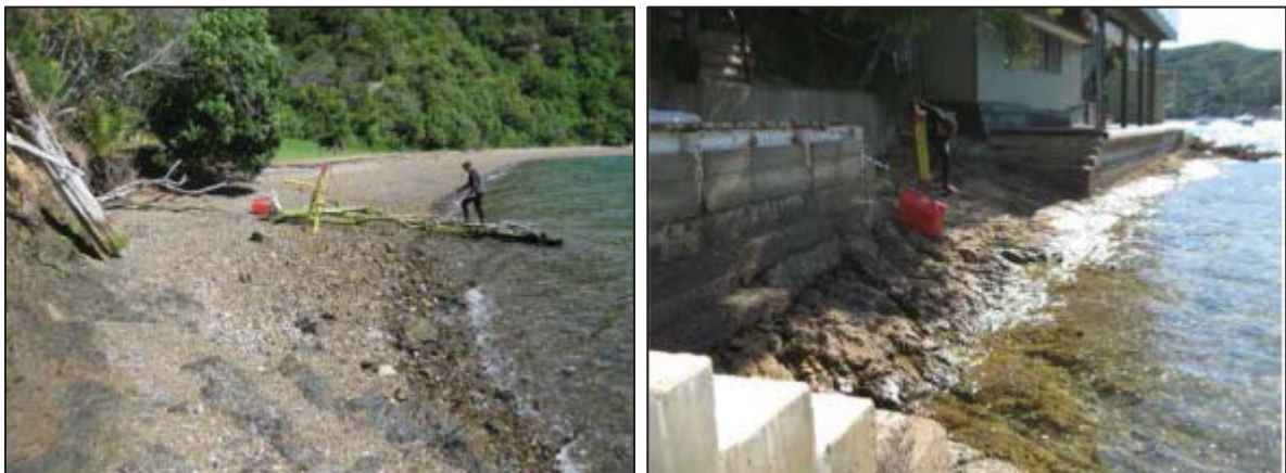
Figure 4 - (Left) Shoreline survey assessment at Bob's Bay (site 8); (Right) Blackmore's in Waikawa (site 5)
