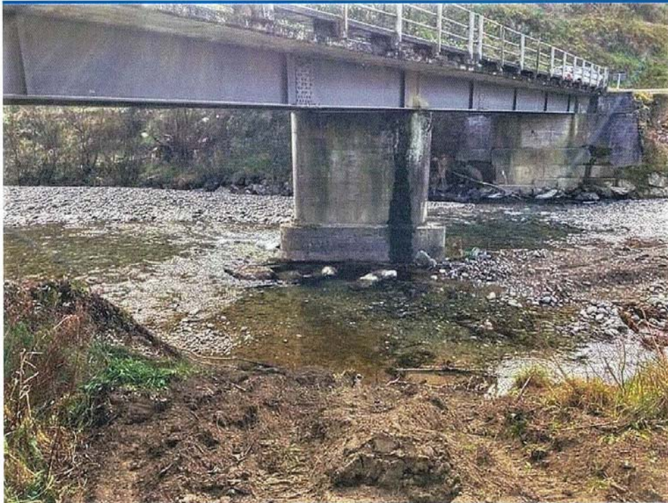
Clearing bridges and culverts on Northbank Road
