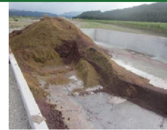
Sealed storage area with leachate collection
