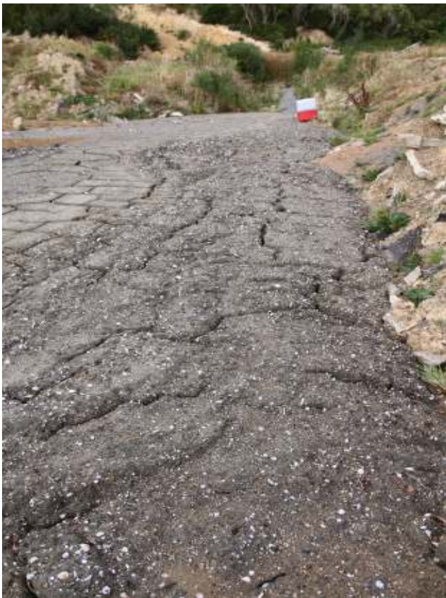
Photo 4: Picton Earthworks. View of the Picton Marine dredged sediments
