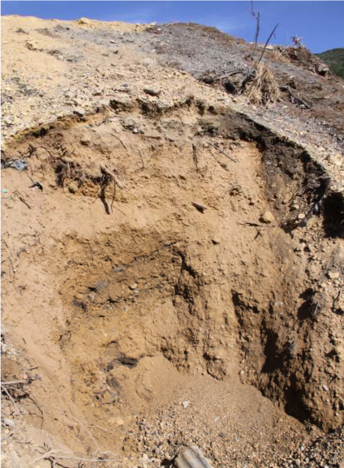
Photo 5: Picton Earthworks. Test Pit 9 typical materials in the tip face
