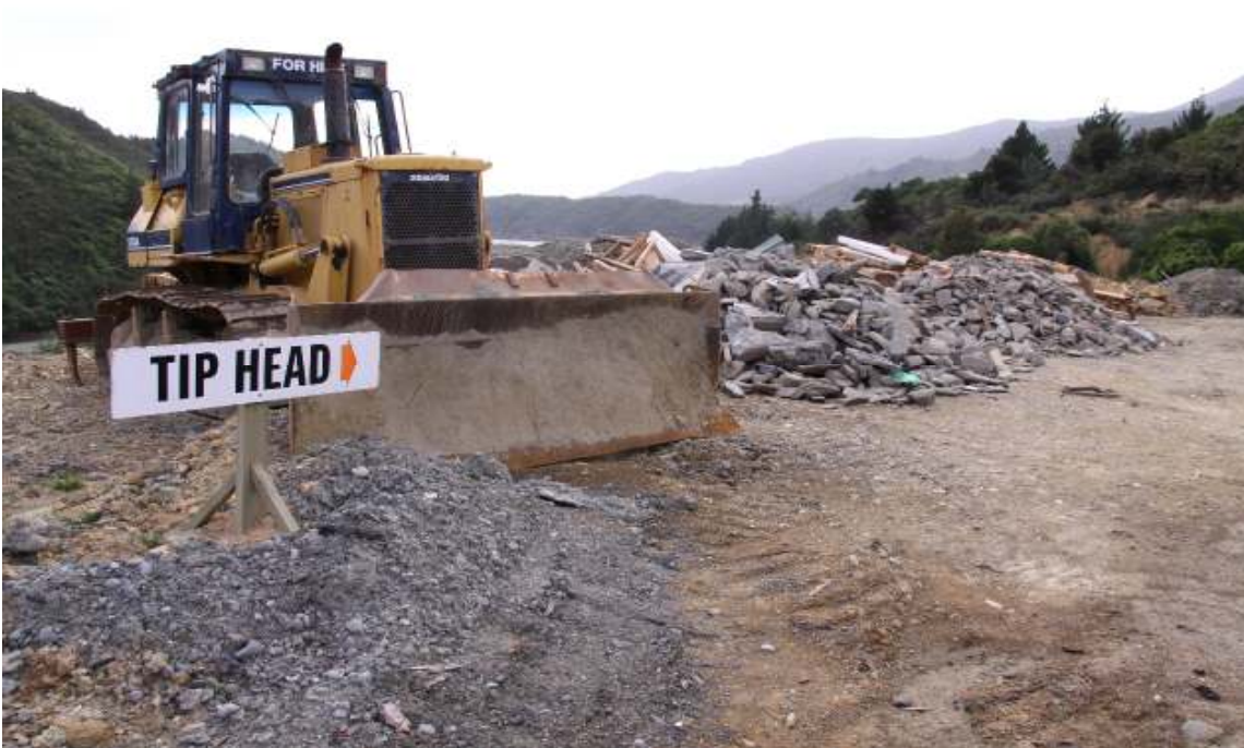
Photo 2: Picton Earthworks. View of materials on the upper platform - tip face
