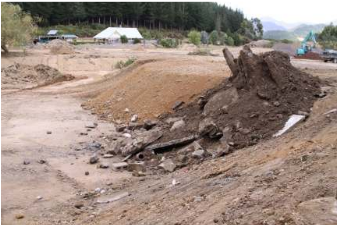
Photo 14: Koromiko Cleanfill Site, Tip Face
