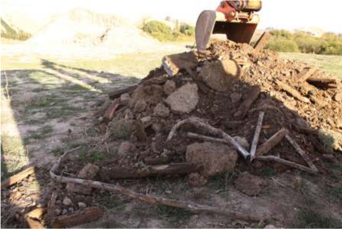
Photo 20: Taylor Pass Road - Test Pit 1 - showing nature of the underlying fill materials
