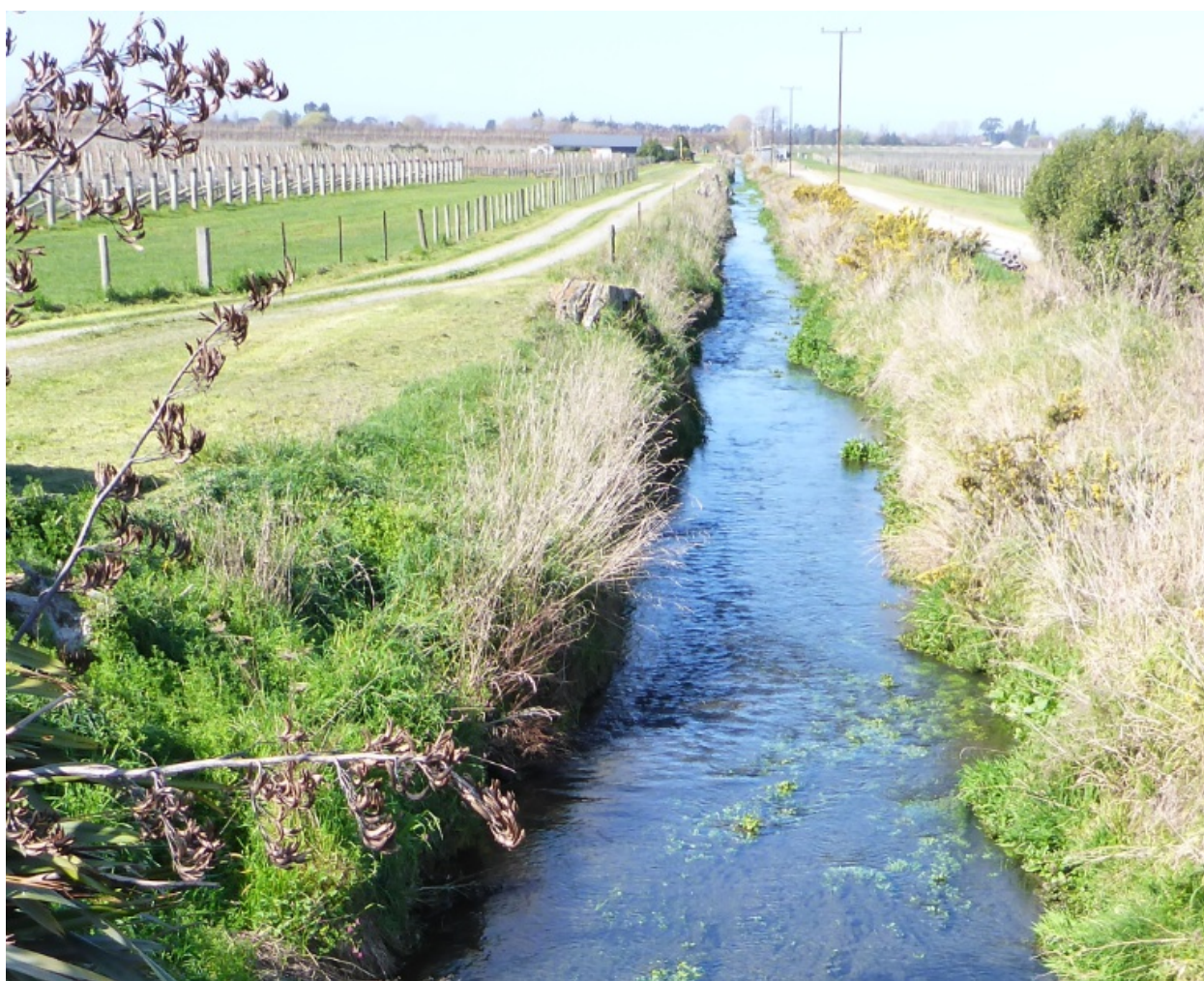
Figure 20: The Fairhall Coop Drain is the largest of the artificial drainage channels constructed in order to lower the groundwater level.
