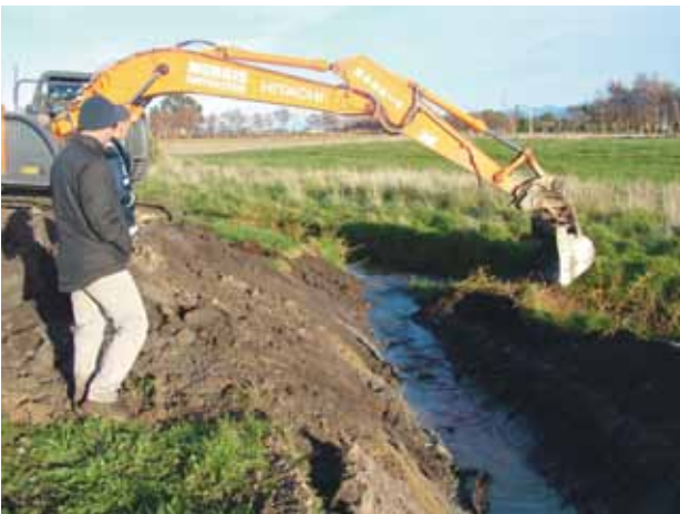
Diverting a waterway
