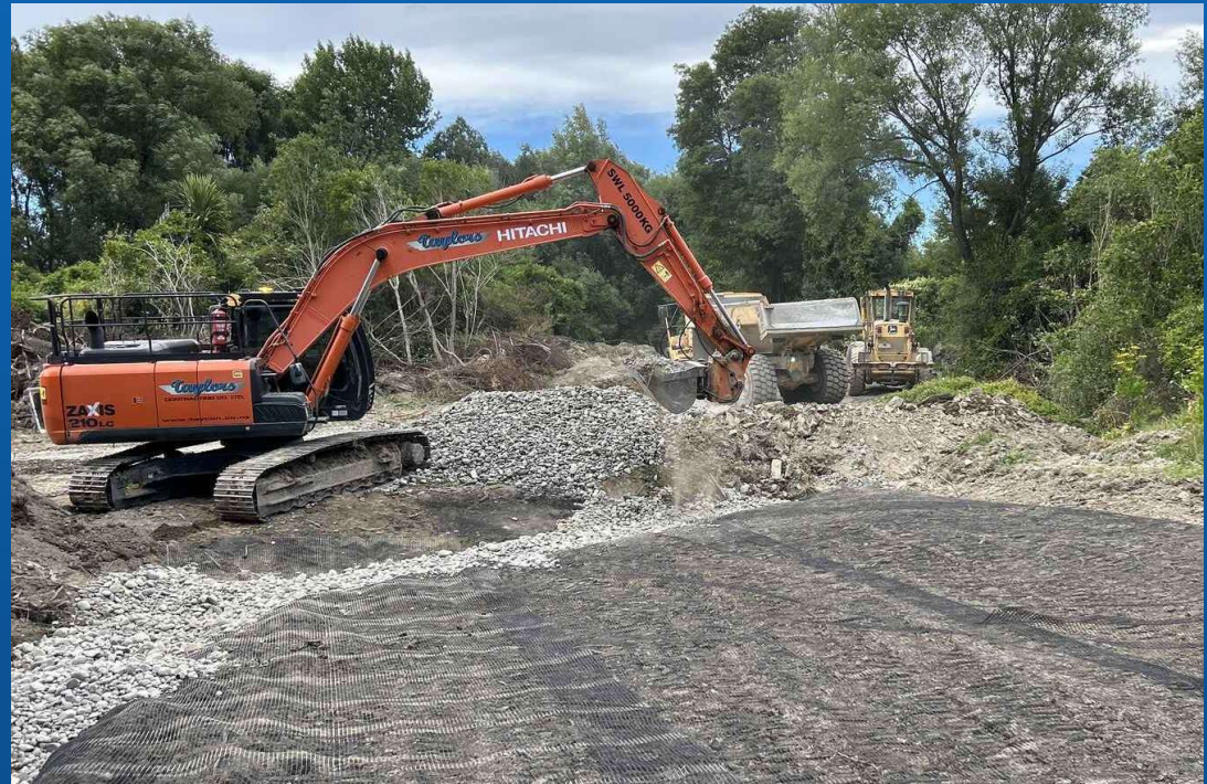
Haul Roads 1,650m of haul road shaped and formed. 13,000 Ton of Gravels used to form roads
