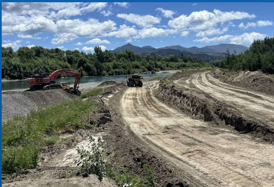
64,000 cube meters of silt and gravel moved
