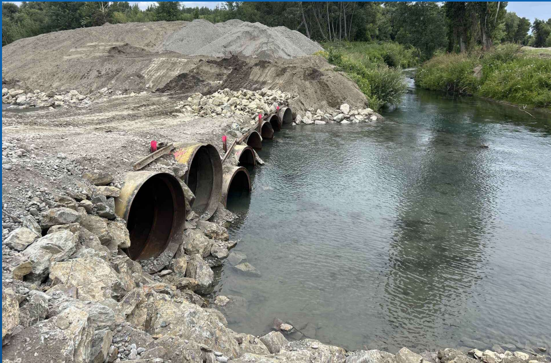
Spring Creek Diversion 8 pipes 2m diameter pipes
