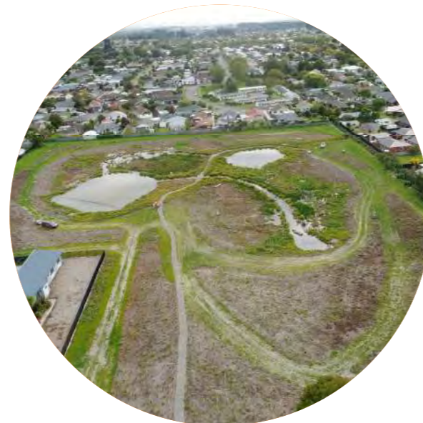
Example: Te Oranga Waikura, Christchurch (Pre plant establishment photo)
