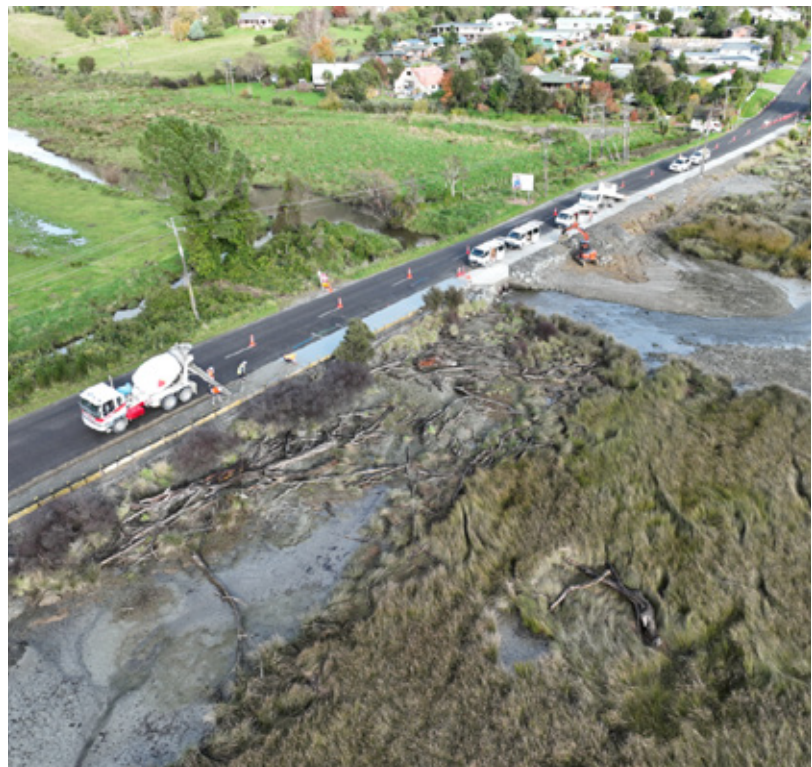
Havelock causeway works in June 2023.
