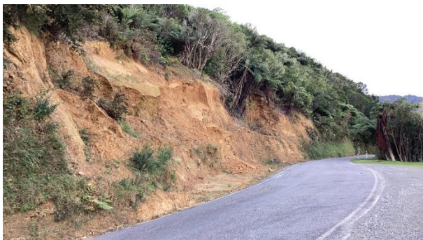
Figure 1-1: Overslip on Anakiwa Road
